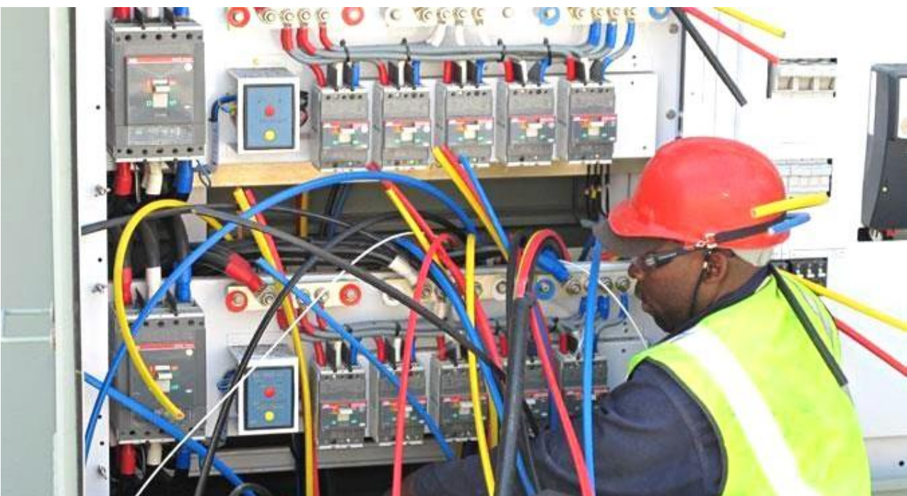
Techmasters' installation of an inverter and batteries.
