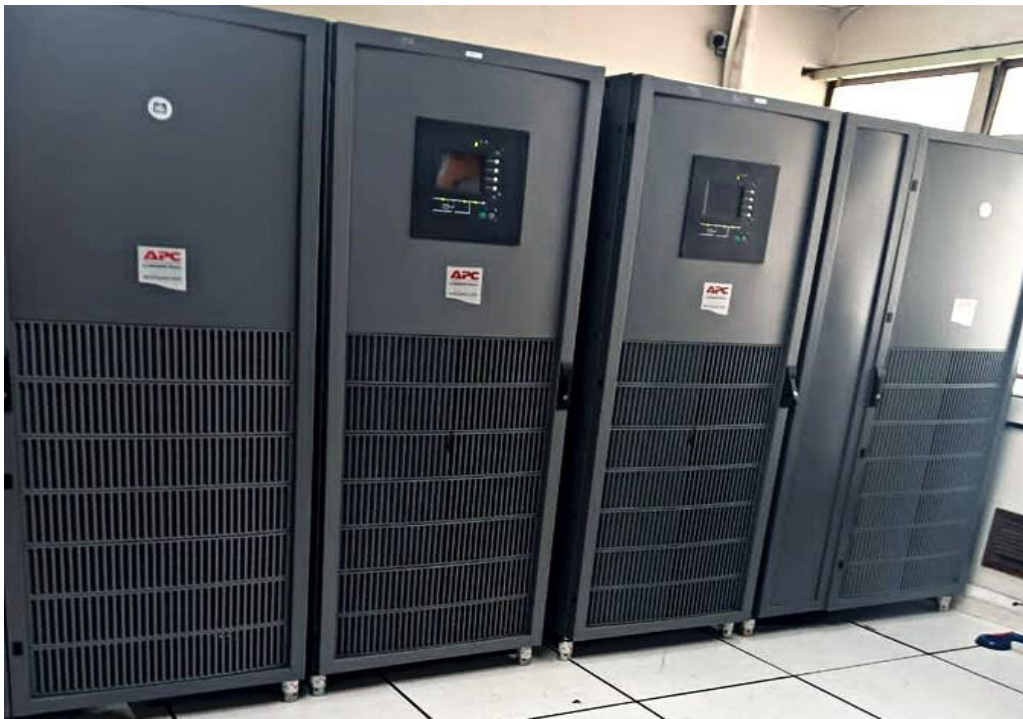
Supply and installation of UPS systems at ZESCO Head Office.
